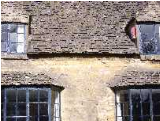
Illustration 31: Stone slates on a High Street cottage – no guttering
