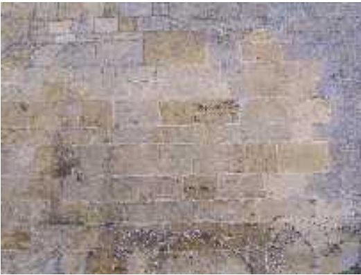
Illustration 36: An example of a "rangework" dressed stone wall
